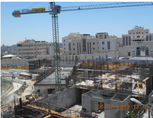
Site progress up to 06 July 2019
