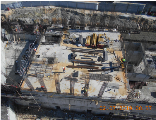
Ground Floor slab cast at block 1
