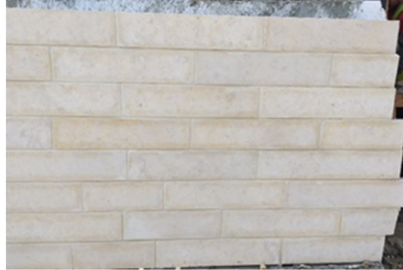
Stone wall mock up done and approved December 2018
