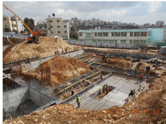
Water tank base reinforcement works at Block 3
