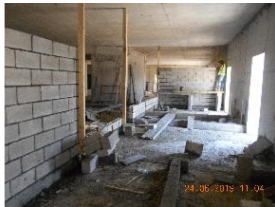
Finishing works started at Basement -2 level
